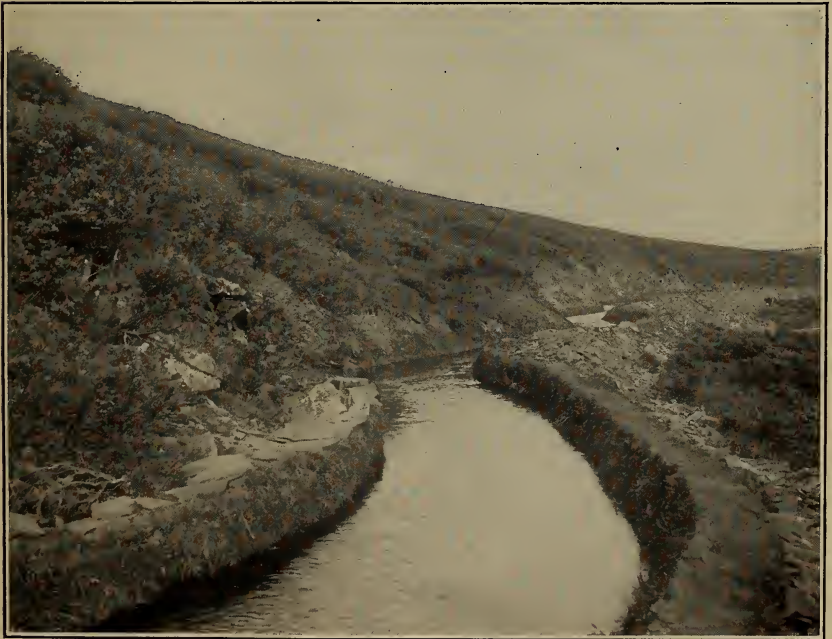
B. HOMESTAKE DITCH, SHOWING SOD WORK.
